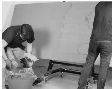
5. BACK BUTTERING OF SLAB
