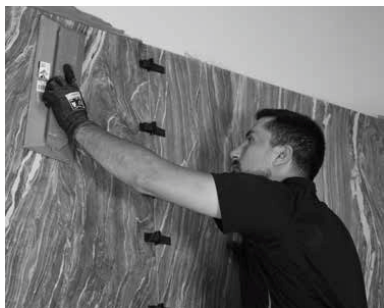
8. SLAB FIXING
